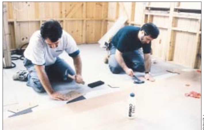
Installing the edge-glued, floating laminate floor is simple enough for the average carpenter — and there's no finishing required.
