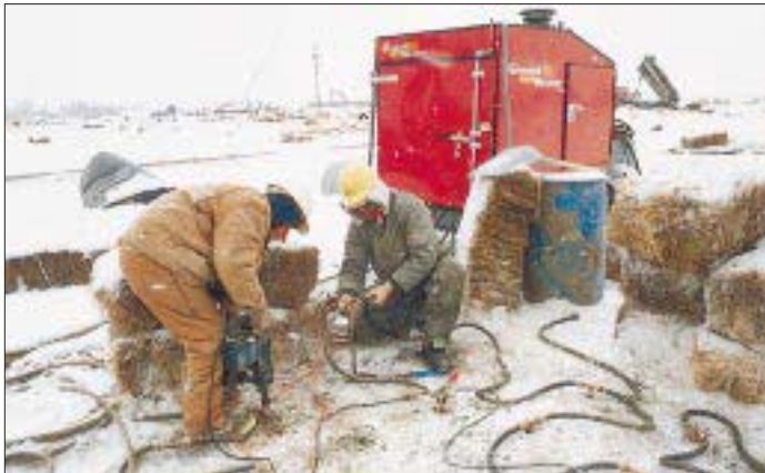
The oil-fired Ground Heater (left) applies heat directly to the earth through rubber tubing, thawing out a foot of frost per day. For deep frost, 3-foot heating probes are inserted into drilled holes (above).
