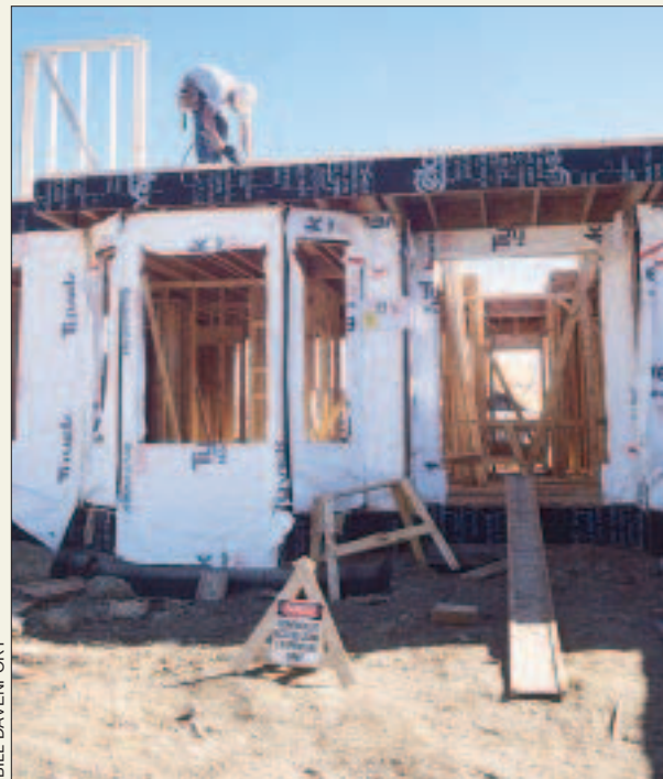
During house framing, fall hazards can't be prevented with scaffolding or tie-offs. Instead, the whole job is designated a "controlled access zone," and only qualified employees who are involved in the work are allowed on the site.
