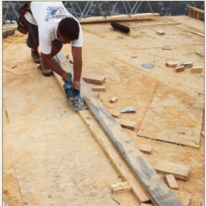
A carpenter rips a long taper using the site-built jig.
