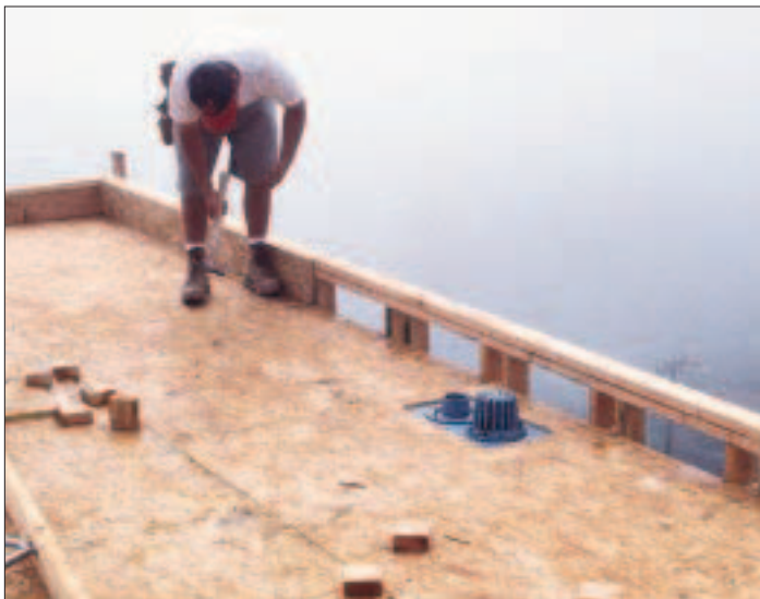
Figure 1. A low parapet wall (left) conceals the slightly pitched roof behind, giving the impression that the roof is perfectly flat. A two-part drain provides for runoff. The main drain, protected by a leaf screen, is plumbed into the home's main waste line; the smaller drain will have an extension to provide backup drainage in case the main drain clogs. The author sometimes places a "cricket" in a corner, to direct ponding water back toward the drain (right).
