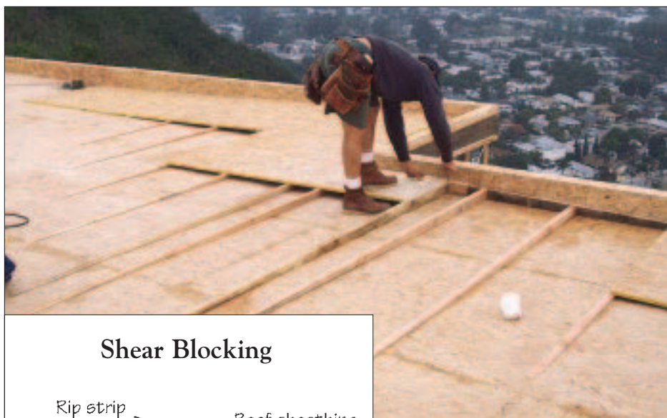
Figure 2. The plans often call for a fully sheathed flat roof to be covered with a second, sloping layer of sheathing (above). On smaller roofs, it is sometimes possible to save the second layer of plywood by nailing the rip strips directly to the rafters. In this case, the engineer may specify full-depth blocking and metal clips over shear walls to ensure transfer of shear forces into the roof diaphragm (left).
