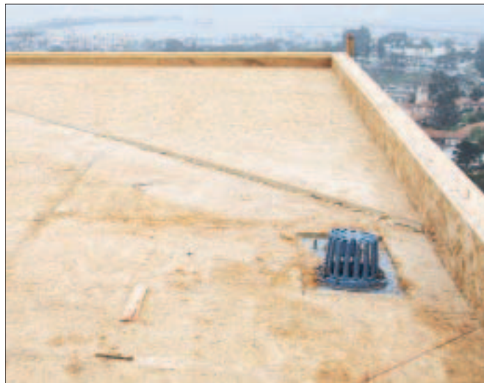
Figure 1. A low parapet wall (left) conceals the slightly pitched roof behind, giving the impression that the roof is perfectly flat. A two-part drain provides for runoff. The main drain, protected by a leaf screen, is plumbed into the home's main waste line; the smaller drain will have an extension to provide backup drainage in case the main drain clogs. The author sometimes places a "cricket" in a corner, to direct ponding water back toward the drain (right).
