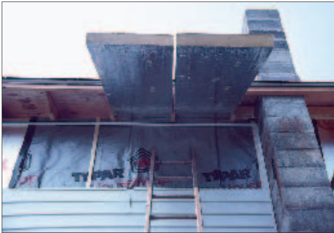
Figure 2. Working from the open eaves, the author slid the snug-fitting rigid foam into place between the I-joists while a worker inside pulled them into place.
