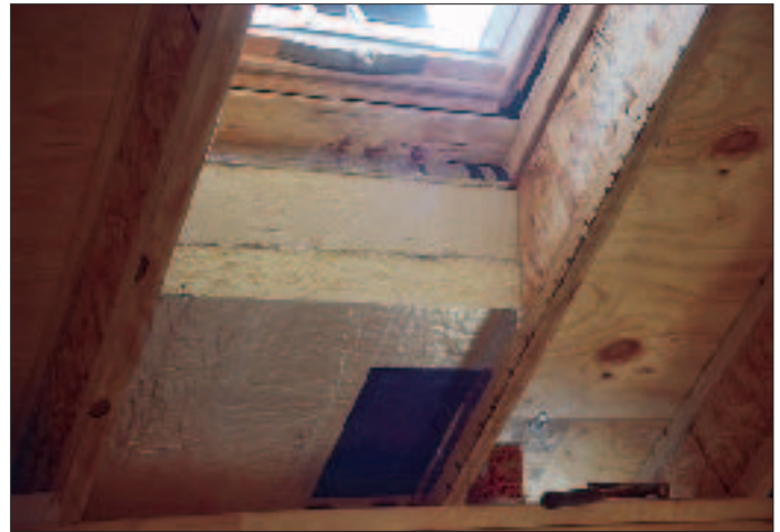
Figure 3. Thin strips of rigid foam inserted above the bottom flange of the I-joists hold the double layer of foam board snug against the top flange. Note the filler piece used to block the vent channel at the skylight well.
