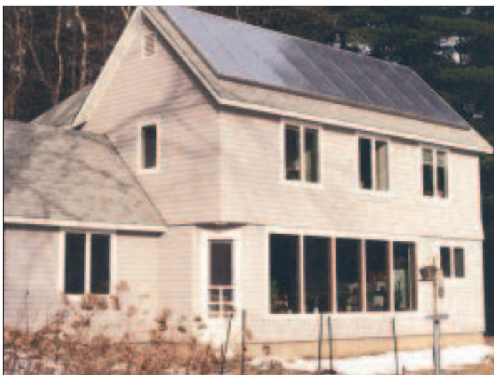
This window wall of 46x76-inch Superglass units has an overall R-value above 7.
