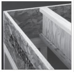
plate — this is not a structural joist. Cost is typically more than for a plywood rim board, but less than for solid wood.
