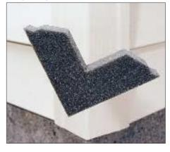
The outside corner trim of a vinyl siding installation makes a great place for bugs to nest. The hollow trim is
