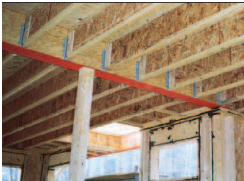
Figure 2. Floor joists laid flush with the top of engineered or steel beams will create a bump in the floor when they shrink (top drawing, left). In these situations, install the joists 1/2 inch high to accommodate the anticipated shrinkage (bottom drawing, left). Where I-joists meet an engineered lumber beam (above), you can install them flush since shrinkage is not an issue with I-joists.
