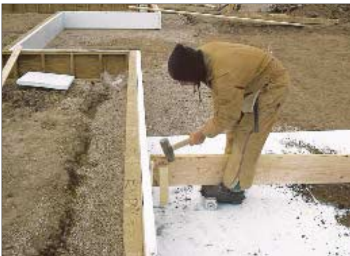
Figure 3. Slabs and footings for unheated buildings, such as the attached garage shown here, are placed directly on top of the foam insulation, with a foot of gravel under the foam. Stakes for the footing forms are driven through the foam (above). A trench is hand-dug inside the perimeter to form the slab's thickened edge (right).
