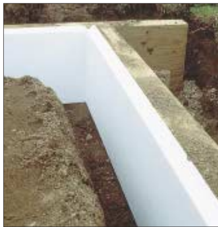
Figure 2. In the photo at left, wooden concrete forms are lined with foam insulation. After the monolithic slab and footing is poured, the forms will be stripped and "wing insulation" placed around the outside perimeter. In the right-hand photo, a permanent wood foundation has foam nailed against it (wing insulation hasn't been added yet). This technique lets the author work in winter: He builds the shell on the wood foundation, then pours the slab.
