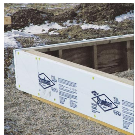
Figure 2. In the photo at left, wooden concrete forms are lined with foam insulation. After the monolithic slab and footing is poured, the forms will be stripped and "wing insulation" placed around the outside perimeter. In the right-hand photo, a permanent wood foundation has foam nailed against it (wing insulation hasn't been added yet). This technique lets the author work in winter: He builds the shell on the wood foundation, then pours the slab.
