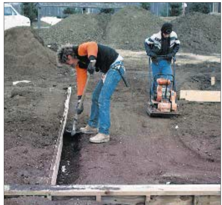
Figure 3. Slabs and footings for unheated buildings, such as the attached garage shown here, are placed directly on top of the foam insulation, with a foot of gravel under the foam. Stakes for the footing forms are driven through the foam (above). A trench is hand-dug inside the perimeter to form the slab's thickened edge (right).
