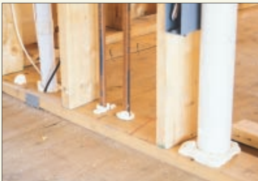
Every hole to the outside should be plugged. Wall penetrations can be sealed with caulk or aerosol foam.
