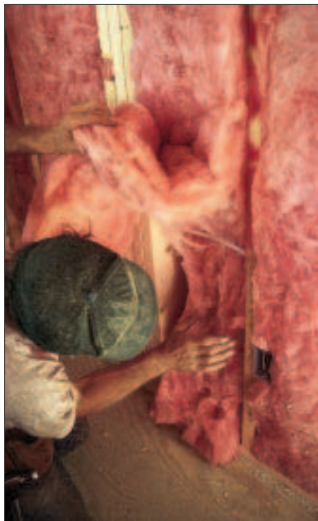
Figure 1. Angles and curves present problems for the fiberglass installer (left). Batts should be split to go around wires, and carefully cut in around electrical boxes (center). Where the budget permits, the author recommends spray-applied foam for insulating odd-shaped cavities (right).
