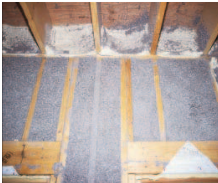
Figure 4. A mix-and-match strategy sometimes provides the builder's best insulation buy. Here, a contractor has used foam to seal up joist bays, window perimeters, and narrow stud bays, while filling most of the wall cavities with spray cellulose.
