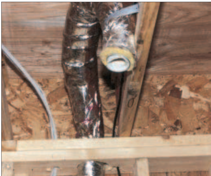
Figure 3. Some situations just can't be handled with fiberglass. Here, wires and ductwork are clogging up the end of a joist bay, making a good fit and good air-seal practically impossible. The author recommends spray foam for such problems.
