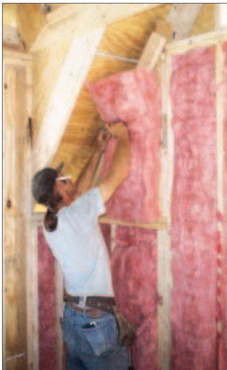
Figure 1. Angles and curves present problems for the fiberglass installer (left). Batts should be split to go around wires, and carefully cut in around electrical boxes (center). Where the budget permits, the author recommends spray-applied foam for insulating odd-shaped cavities (right).
