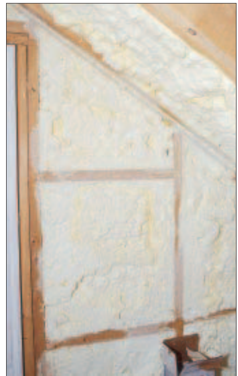
Figure 1. Angles and curves present problems for the fiberglass installer (left). Batts should be split to go around wires, and carefully cut in around electrical boxes (center). Where the budget permits, the author recommends spray-applied foam for insulating odd-shaped cavities (right).
