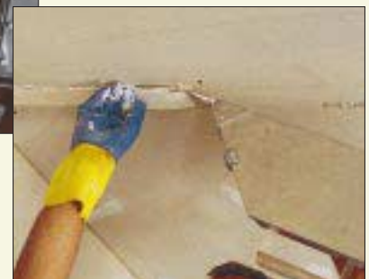
A taping banjo makes quick work of bedding drywall tape. You fill the mud compartment (above), and the tape is coated with compound as it's pulled from the banjo (right).
