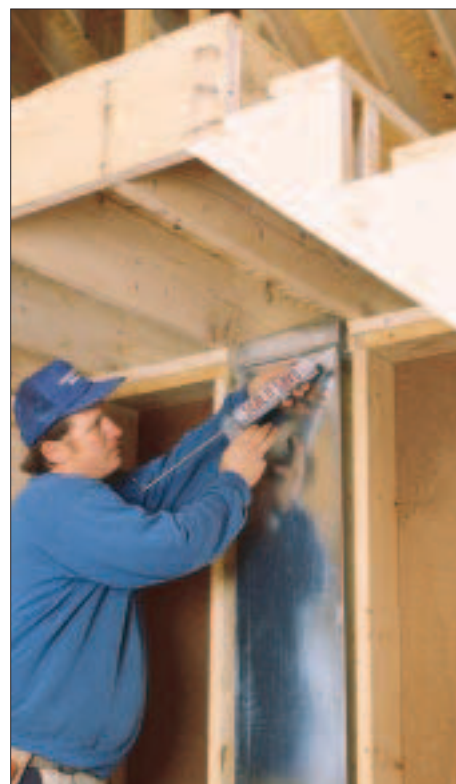
Figure 2. Air systems usually leak at joints between branch ducts and the main trunk line and at the connections between supply ducts and registers (left). Replace all duct tape with mesh tape and a high-quality mastic. Pay close attention to sealing cracks where ductwork penetrates unconditioned spaces such as attics or basements (right).
