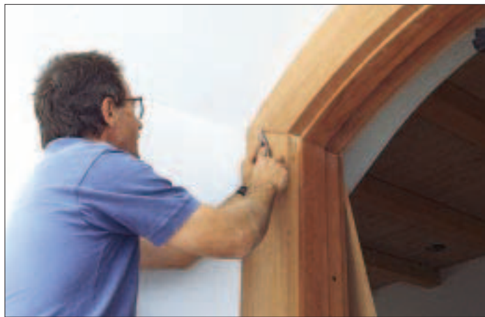
Polyurethane glues foam and expand as they set, helping to fill gaps in the joints (left). The squeeze-out can be cleaned immediately with mineral spirits, but the author prefers to use a chisel on the excess after it has dried (right).
