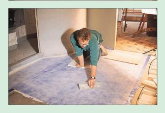
liquid and smoothed into place with trowels, taping knives, or other tools. Specific instructions may call for additional coats of liquid to complete the installation. Although this type of membrane is not my usual choice for waterproofing or crack isolation, it may be the most practical choice when you are faced with waterproofing a complex area like a set of stairs leading into a tub or pool.
