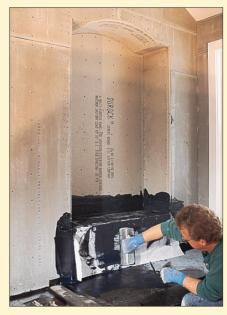
First, a thick liquid is poured on the tile backerboard and troweled into place (left), followed by a fiberglass or polyester reinforcing fabric (center). The author then laps the fabric up walls and around corners, smooths it into place with a trowel, and follows with a second coat (right). This approach works well for waterproofing complex areas like stairs leading up to a tub.
