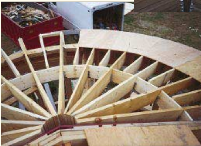
To support a round roof without collar ties, the author designed a radial rafter system (left) supported by a custom steel "girder truss" (above).
