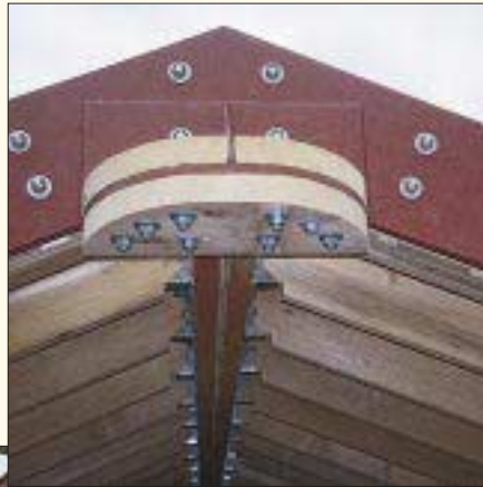
To support a round roof without collar ties, the author designed a radial rafter system (left) supported by a custom steel "girder truss" (above).
