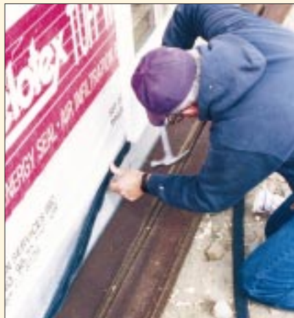
A strip of folded screening in the lower opening keeps wasps and bees from nesting behind the siding.
