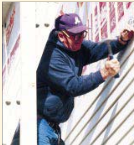
Builder Lud Leskovar uses pre-primed siding and takes care to prime each cut end. The pre-primed siding has a good appearance as soon as it's installed, he notes.
