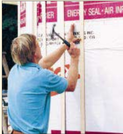
Carpenters nail furring strips over the housewrap to create an air space behind clapboards.
