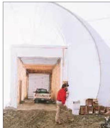
Inside the structure, the Roundtree Construction crew works in comfort (left). At right, a truck exits through the airlock tunnel.
