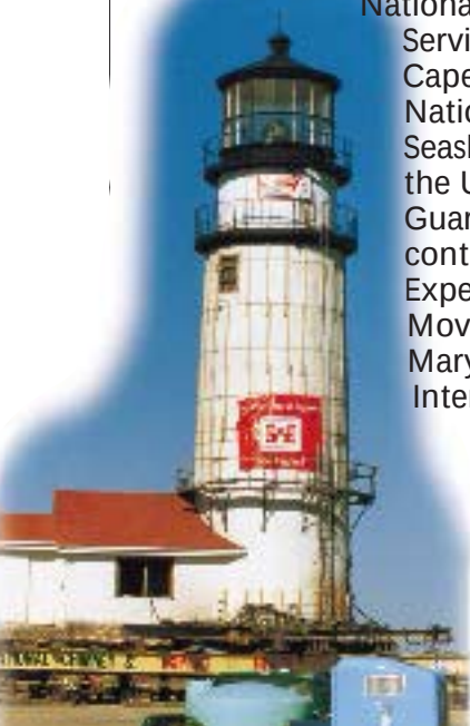
Cape Cod's Highland Light being "corseted" and placed on a system of support beams in preparation for a five-day, 150-yard move west.
