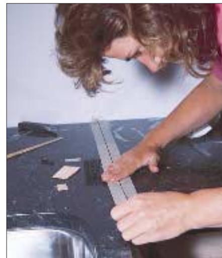
The finishing touches: Aikey carefully preps a joint between two counter runs for sealing.
