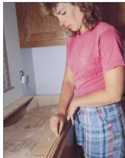
Anita Aikey measures a template for a sink in a counter of Verde Antique marble. "About the worst thing you can do," she says, "is mess up that template. I try to take my time with those."
