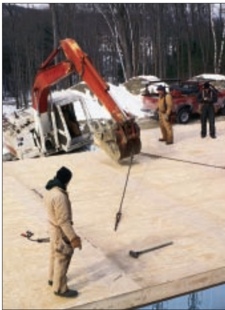
Figure 3. Once the floor system is assembled, it may need to be shifted slightly on the foundation. The author uses his excavator to push or pull the floor into place, but come-alongs chained to a tree will get the job done.
