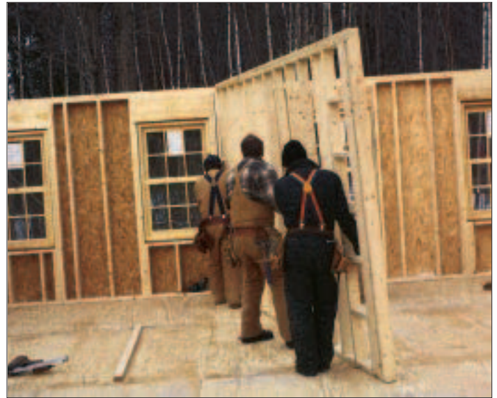
Figure 4. Exterior walls drop into place as the lead man lays out the interior (left). Interior walls are boomed into the house in bundles and hand-carried into place (right).
