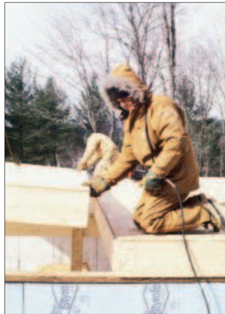
Figure 2. The author's crew lays down an entire floor deck in about an hour. The first panel is set as straight as possible (top), then a carpenter lays a bead of construction adhesive on the exposed edge of the last joist (left center). The next panel is set alongside (right center), and the two panels are pulled tightly together with come-alongs. A carpenter nails the panels together at the plywood joint (left).
