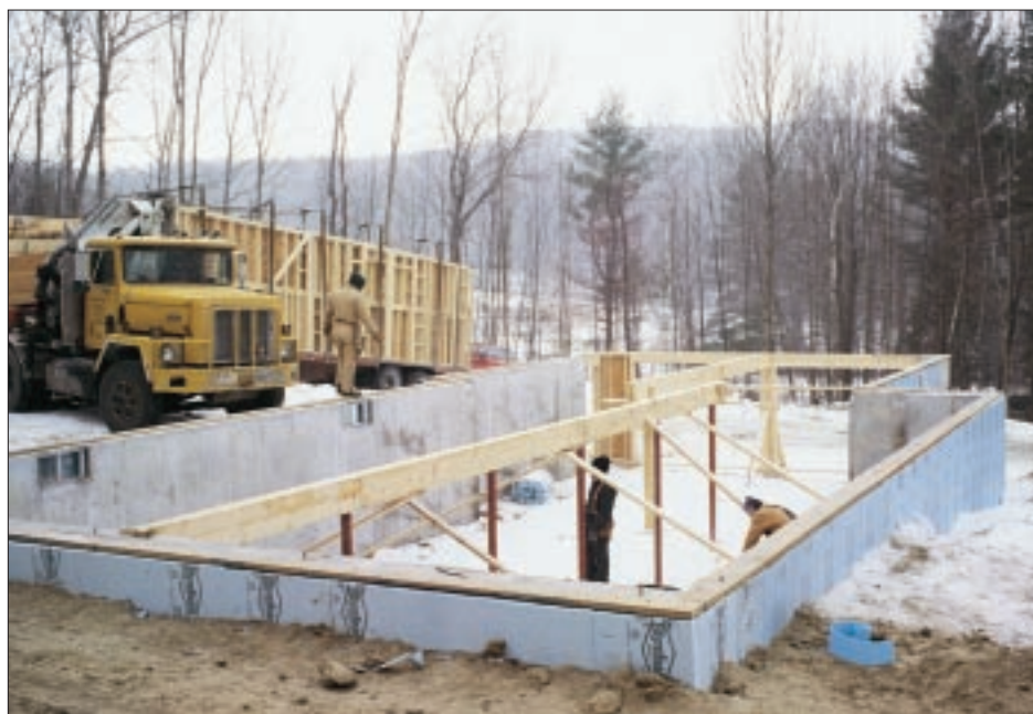
Figure 1. With sills and girders in place, the foundation is ready for the house package. Everything from housewrap to skylights arrives on the boom trucks.
