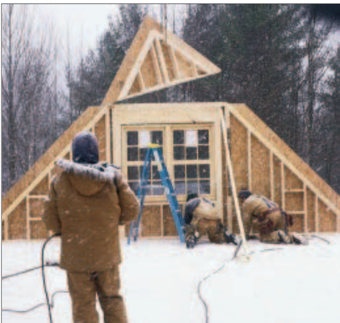
Figure 5. Gable walls go as quickly as any other element of the package. With his remote control, the crane operator has a clear view of the job.
