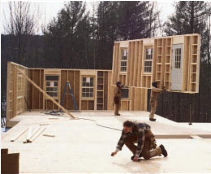
Figure 4. Exterior walls drop into place as the lead man lays out the interior (left). Interior walls are boomed into the house in bundles and hand-carried into place (right).
