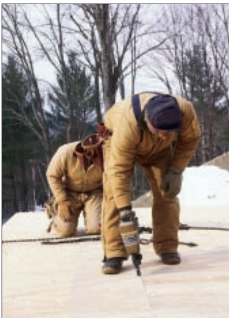
Figure 2. The author's crew lays down an entire floor deck in about an hour. The first panel is set as straight as possible (top), then a carpenter lays a bead of construction adhesive on the exposed edge of the last joist (left center). The next panel is set alongside (right center), and the two panels are pulled tightly together with come-alongs. A carpenter nails the panels together at the plywood joint (left).
