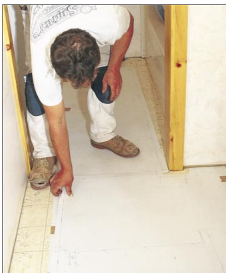
Figure 2. To ensure a perfect fit, pattern paper is laid over the entire floor area (left). Then the outlines of the room perimeter, as well as doorways, cabinets, and other obstructions, are scribed onto the paper using a steel square (center). In the shop, the markings are transferred to the sheet flooring (right) and cut with a knife against a straightedge.
