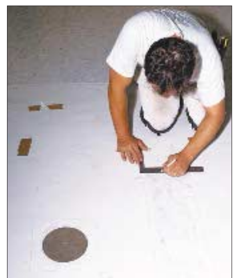
Figure 2. To ensure a perfect fit, pattern paper is laid over the entire floor area (left). Then the outlines of the room perimeter, as well as doorways, cabinets, and other obstructions, are scribed onto the paper using a steel square (center). In the shop, the markings are transferred to the sheet flooring (right) and cut with a knife against a straightedge.
