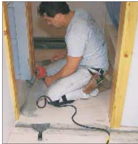
Figure 1. For underlayment, the author prefers to use \frac{3}{8} - or \frac{1}{2} -inch PTS plywood or Type 1 lauan, fastened with 1\frac{1}{8} -inch galvanized staples (left). A cementitious compound recommended by the flooring manufacturer is mixed with latex and used to fill all joints (above).
