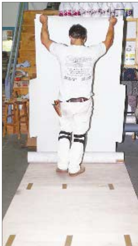
Figure 3. The author prefers to install his own underlayment. After taping together rough-cut sheets of plywood laid on the shop floor (left), he traces the outline of the finished flooring on top and cuts the plywood to size.
