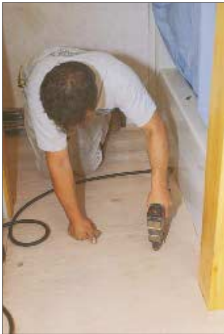
Figure 1. For underlayment, the author prefers to use \frac{3}{8} - or \frac{1}{2} -inch PTS plywood or Type 1 lauan, fastened with 1\frac{1}{8} -inch galvanized staples (left). A cementitious compound recommended by the flooring manufacturer is mixed with latex and used to fill all joints (above).
