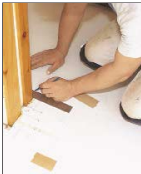
Figure 2. To ensure a perfect fit, pattern paper is laid over the entire floor area (left). Then the outlines of the room perimeter, as well as doorways, cabinets, and other obstructions, are scribed onto the paper using a steel square (center). In the shop, the markings are transferred to the sheet flooring (right) and cut with a knife against a straightedge.
