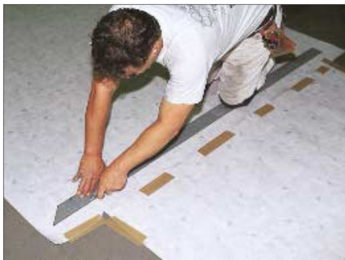
Figure 4. When cutting seams in thin flooring material, the meeting edges are overlapped and cut at the same time. Thicker sheets are cut separately and butted.
