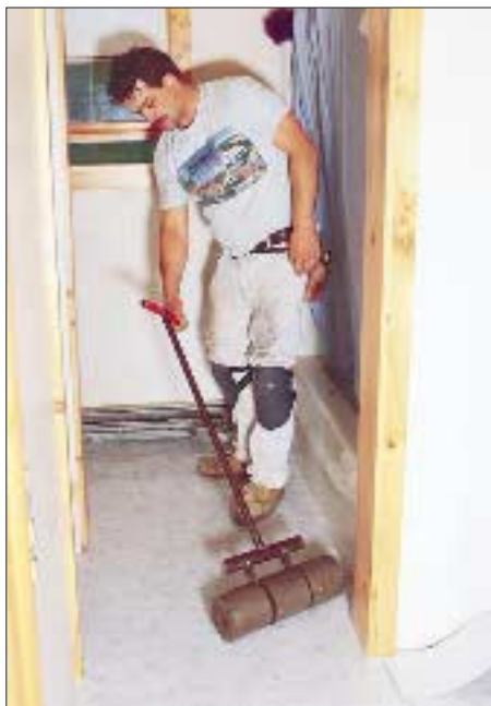
Figure 5. Edges that can't be covered with molding are epoxied in place using a special edging tool and a hand roller (left). The entire floor is pressed into the adhesive with a 150-pound roller (right).
