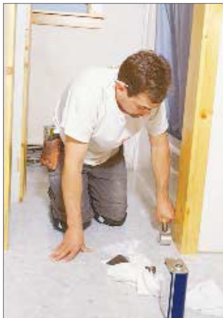
Figure 5. Edges that can't be covered with molding are epoxied in place using a special edging tool and a hand roller (left). The entire floor is pressed into the adhesive with a 150-pound roller (right).
