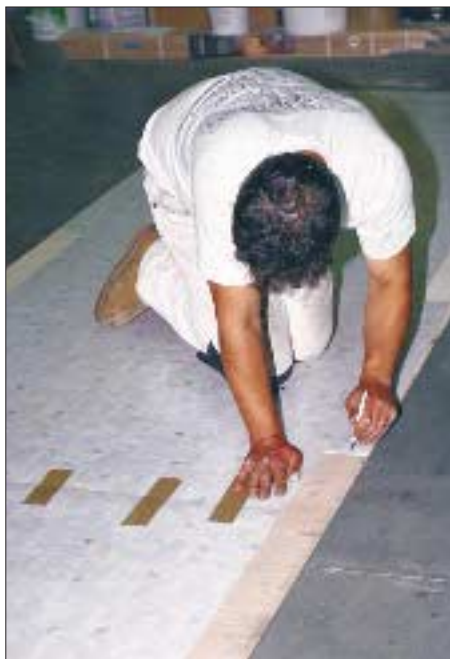
Figure 3. The author prefers to install his own underlayment. After taping together rough-cut sheets of plywood laid on the shop floor (left), he traces the outline of the finished flooring on top and cuts the plywood to size.
