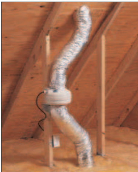
Figure 1. In-line fans are mounted in the attic (shown) or basement, between a grille in the bathroom and the outside wall jack. The insulated duct helps reduce sound transmission and prevents condensation.
