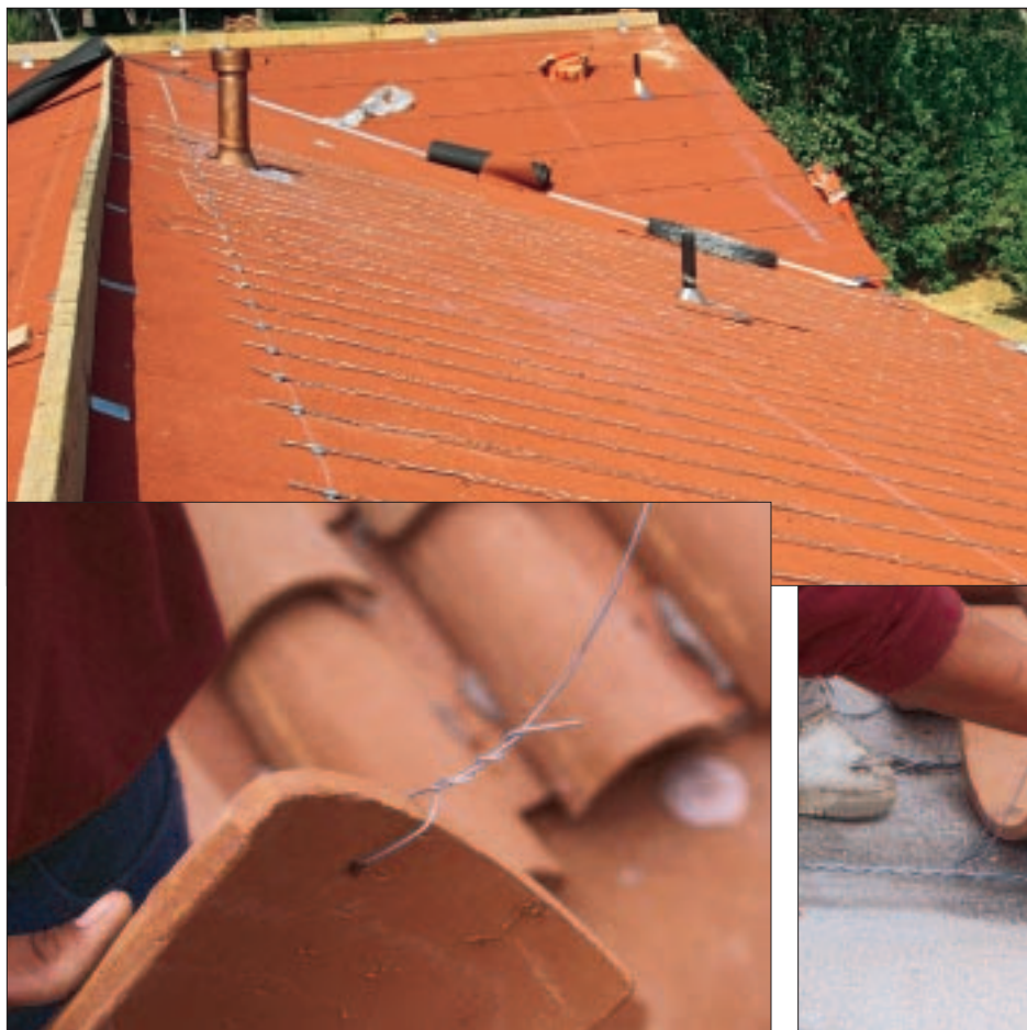
Figure 3. The twisted-wire method uses a double strand of 14-gauge wire fastened at the ridge and eaves with special anchors (left). Each tile is secured with an individual tie wire (below left) that is threaded through the open loops in the twisted wire (below).
