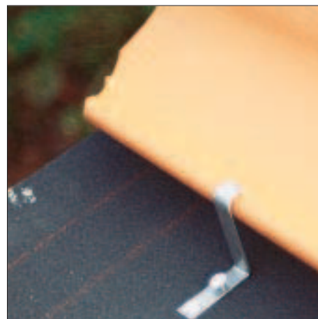
Figure 4. Nose clips (left) hold down the front end of the tile. The same nail secures both the nose clip and the tile underneath. Hurricane clips (right) are L-shaped brackets that hook over the side of a roof tile. According to the author, these clips have a tendency to deform and work loose in repeated winds, so should only be used as backup protection.
