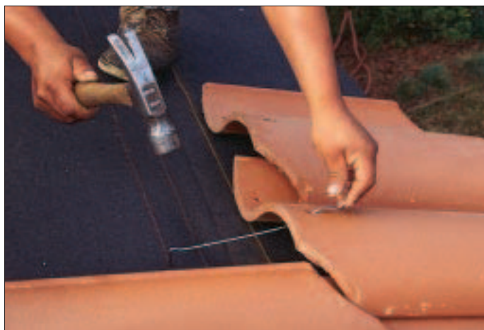
Figure 4. Nose clips (left) hold down the front end of the tile. The same nail secures both the nose clip and the tile underneath. Hurricane clips (right) are L-shaped brackets that hook over the side of a roof tile. According to the author, these clips have a tendency to deform and work loose in repeated winds, so should only be used as backup protection.
