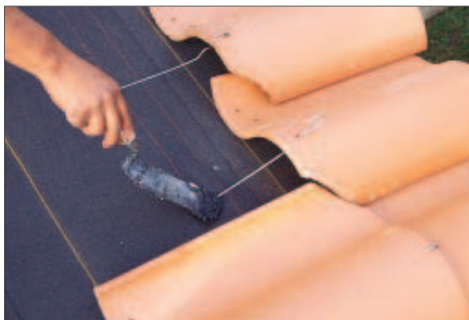
Figure 5. The Tile Nail from Newport Fasteners has several advantages over a conventional nose clip. Because it is driven in a few inches away from the tile (above left), there is less risk of cracking the tile while nailing. Its length allows enough movement to keep the tile from breaking during high winds or an earthquake. Also, the nail holes can be patched with mastic to prevent leaks in the membrane (left).
