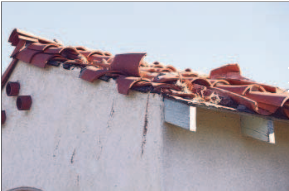
Figure 1. Mortar systems are popular because they don't penetrate the underlying waterproof membrane with nails. Unfortunately, they are also prone to destruction from high wind, as evidenced by the eaves damage on this house.
