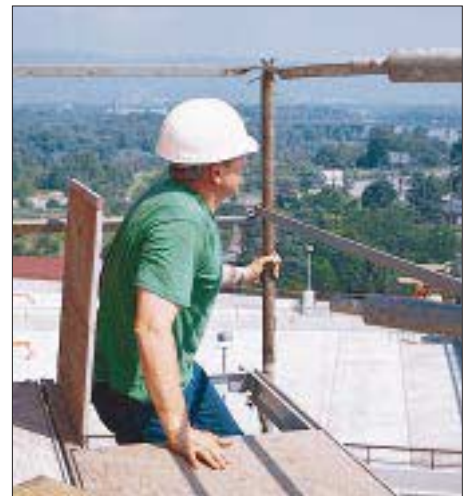
Figure 3. Manufactured platforms are available with hatches that allow workers to reach the work area from within the scaffold framing system.
