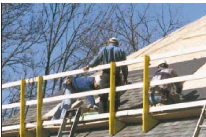
Figure 7. E-Z Rail roof brackets are designed to provide an OSHA-approved guardrail system.
