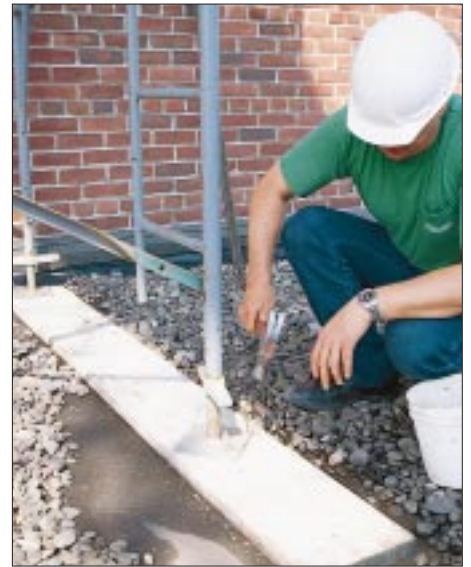
Figure 1. Always set tubular steel scaffolding on a steel base plate on top of level wood sills. Tack the bases to the wooden sills with 10d nails.
