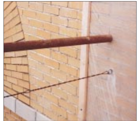
Figure 2. When tying scaffolding to masonry structures, use a tubular tie-in in conjunction with an eyebolt. The author recommends a vertical tie-in spacing of no more than four times the smallest base dimension.
