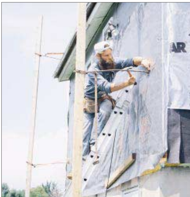
Figure 5. Pump-jack poles require intermediate bracing every 10 feet. Installing an additional pole bracket is the easiest way to provide this bracing.
