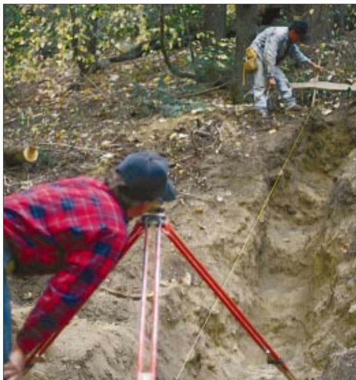
Figure 1. Using a plumb bob, the author positions his transit over the intersection of his first two strings (left). Then he sights down the second string to establish a 90-degree corner (right). A helper fastens the end of the string in place.
