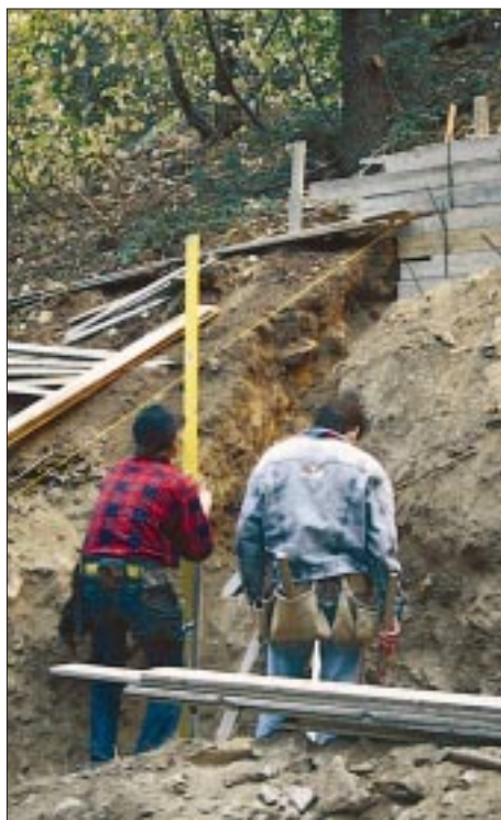
Figure 2. Using the strings as a guide, carpenters plumb the stakes to the line (left). After the forms are nailed together (center), they plumb and brace the wall section (right).
