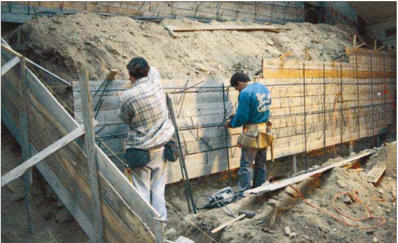
Using rough-sawn 1x6, the author can form anything from high retaining walls to complicated stemwall systems.
