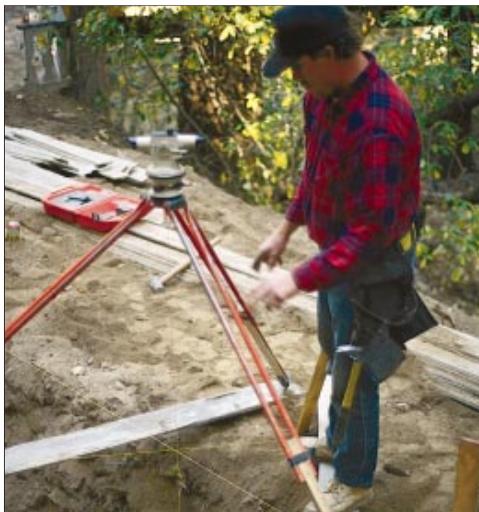
Figure 1. Using a plumb bob, the author positions his transit over the intersection of his first two strings (left). Then he sights down the second string to establish a 90-degree corner (right). A helper fastens the end of the string in place.
