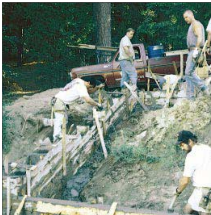
Figure 4. The author uses strips of \frac{3}{4} -inch plywood for the bulkheads that form the vertical steps in a stemwall.
