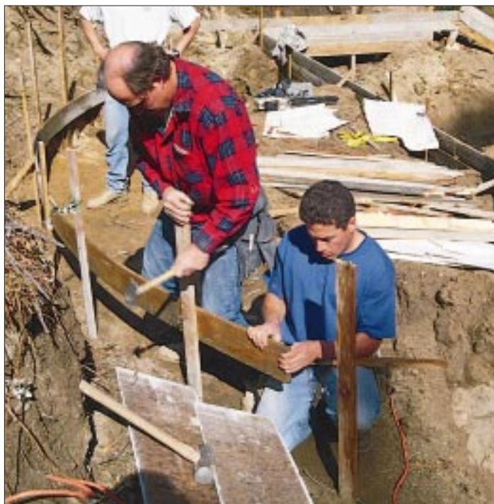
Figure 3. Odd angles and even curves are easy with this forming method. For curves, the boards bend more easily if they're wet.
