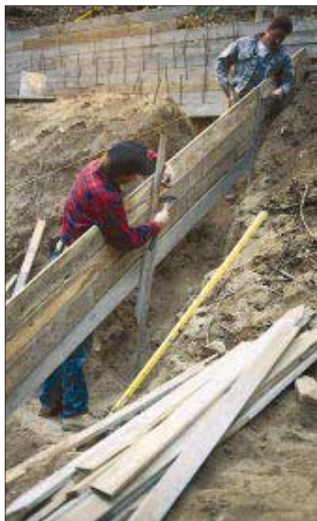
Figure 2. Using the strings as a guide, carpenters plumb the stakes to the line (left). After the forms are nailed together (center), they plumb and brace the wall section (right).
