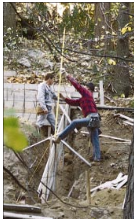
Figure 2. Using the strings as a guide, carpenters plumb the stakes to the line (left). After the forms are nailed together (center), they plumb and brace the wall section (right).
