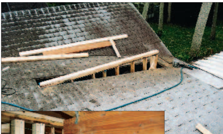
Figure 2. Short kneewalls built on top of first-floor bearing walls support the addition (left). To avoid exposing the lower story to the weather, the carpenters opened only as much of the roof as necessary to frame the kneewalls (above).
