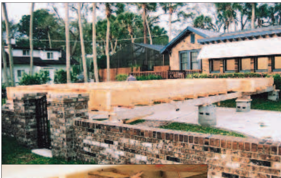
Figure 1. The author's crew framed the 32x18-foot addition on built-up beams supported on cement block piers (above). Hangers attached to the floor joists held the steel I-beams used to lift the addition (left).
