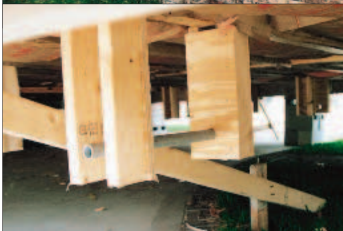
Figure 1. The author's crew framed the 32x18-foot addition on built-up beams supported on cement block piers (above). Hangers attached to the floor joists held the steel I-beams used to lift the addition (left).
