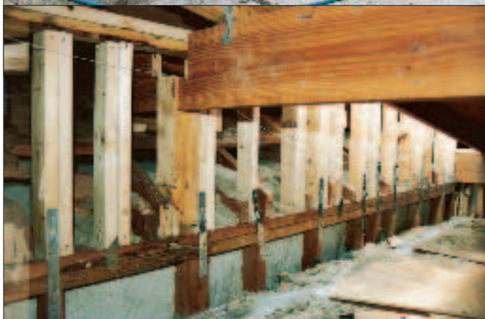
Figure 2. Short kneewalls built on top of first-floor bearing walls support the addition (left). To avoid exposing the lower story to the weather, the carpenters opened only as much of the roof as necessary to frame the kneewalls (above).
