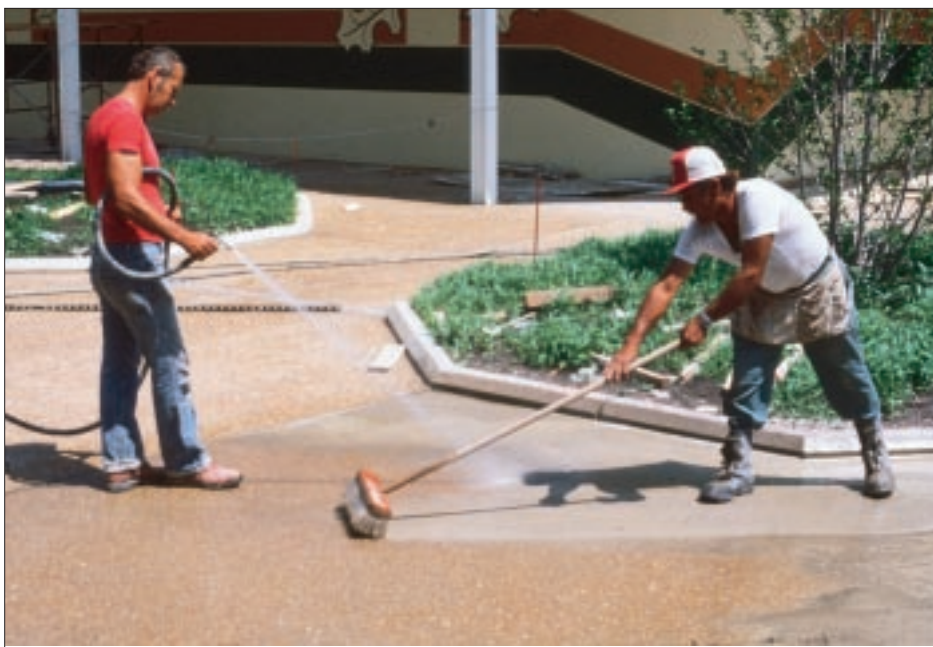
Figure 5. It takes two people to expose the aggregate in a slab. A broom is used to “pull off” the cement paste that accumulates ahead of the spray.
