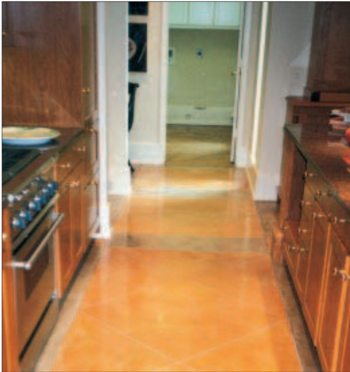
Figure 2. Surface stains, tooling, and polishing can give a concrete slab the look of expensive marble.
