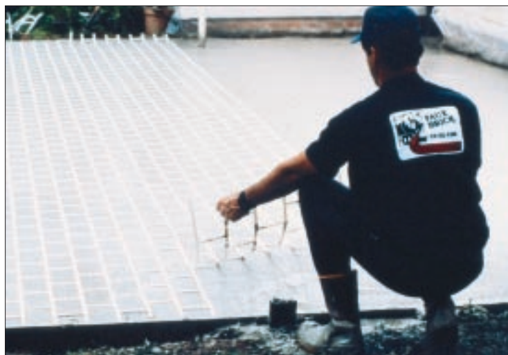
Figure 3. Repetitive patterns can be pressed into the surface of freshly poured concrete using stamps (left) or plastic templates (right).
