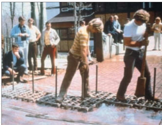
Figure 3. Repetitive patterns can be pressed into the surface of freshly poured concrete using stamps (left) or plastic templates (right).
