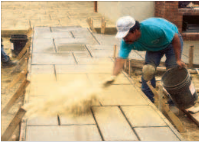
Figure 1. With the “dry shake” method, a powdered dye is broadcast over the surface of the slab, then troweled in.
