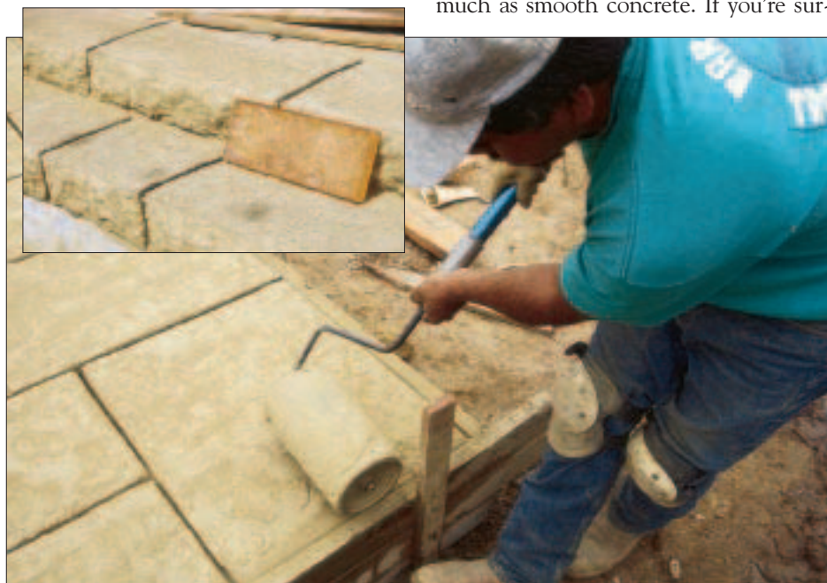
Figure 4. Pattern rollers can create the look of smooth pavers or natural stone. Here, the stone texture on the surface of the concrete is matched on the edges of the steps by using molded rubber form liners (inset).
