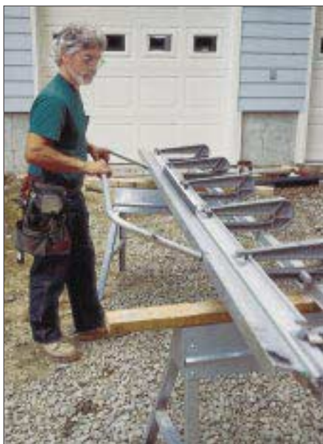
The author bends all the flashings for the additions he builds using a refurbished second-hand brake.
