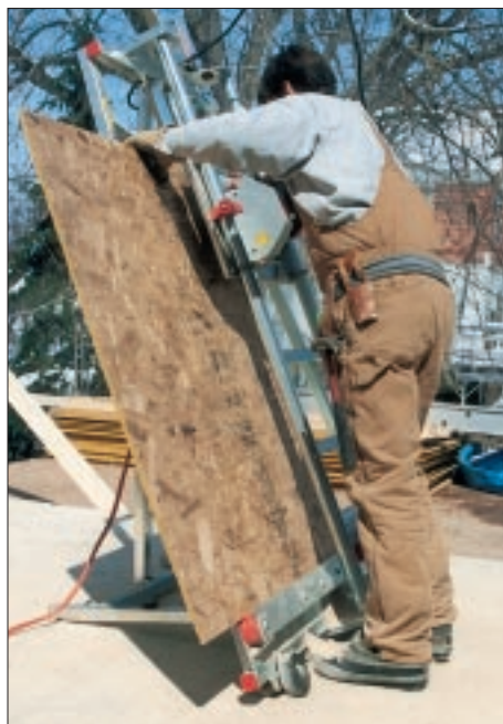
Figure 1. The author hauled his SSC C-4 panel saw up to the second-floor roof deck to cut wall and roof sheathing.
