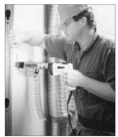
Using the Rocker, a worker can drive the 50 screws on the flat plastic tape just as fast as he can find the right spot and push. This increased production can help offset the investment in the tool.
