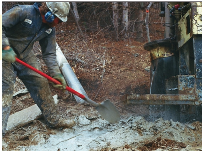
The drill operator directs the slurry of rock fines and water away from the hole.
