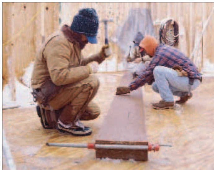
Figure 2. Clamps help with alignment when nailing or bolting together a built-up LVL beam.
