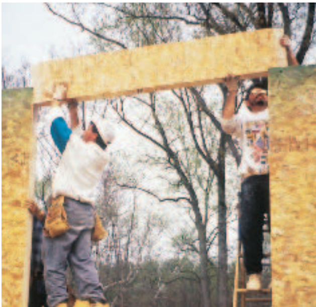
Figure 4. For heavy loading, structural headers slip into recessed pockets in the wall panels. Trimmer studs are embedded in the panel by the panelizer.
