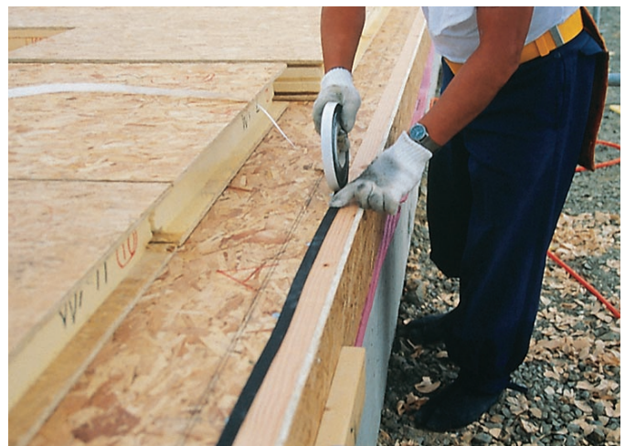
Figure 2. Just like stick-framed walls, panel walls are assembled on the deck, then lifted into place (left). The foam in the bottom of the panel is recessed to slip over a bottom plate, which is first mounted on the perimeter of the floor deck. Here, a worker installs an air-seal gasket just before the wall is stood up (right).
