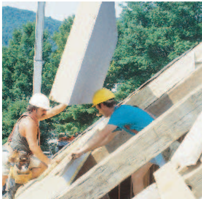
Figure 5. Roof panels may be supported by rafters spanning from ridge to eaves (left), or by purlins set into gable walls (above). A post in the gable panel below the purlin may or may not be necessary, depending on the calculated roof loads.
