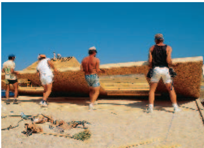
Figure 2. Just like stick-framed walls, panel walls are assembled on the deck, then lifted into place (left). The foam in the bottom of the panel is recessed to slip over a bottom plate, which is first mounted on the perimeter of the floor deck. Here, a worker installs an air-seal gasket just before the wall is stood up (right).
