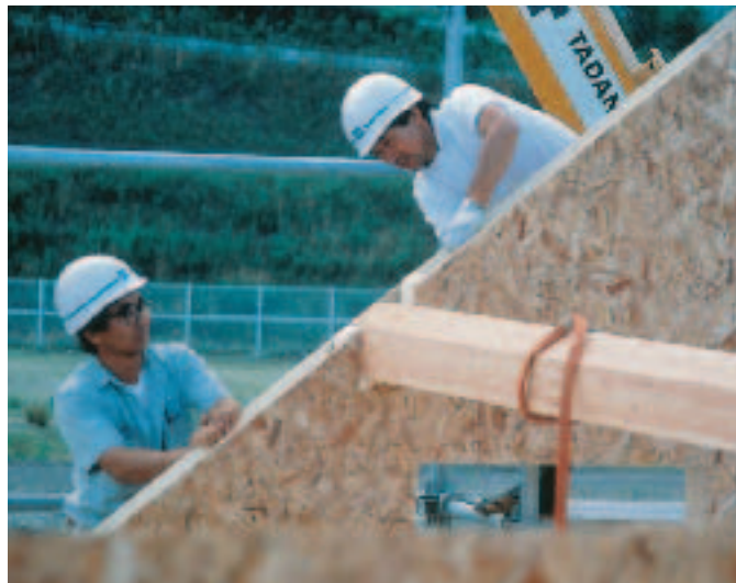
Figure 5. Roof panels may be supported by rafters spanning from ridge to eaves (left), or by purlins set into gable walls (above). A post in the gable panel below the purlin may or may not be necessary, depending on the calculated roof loads.
