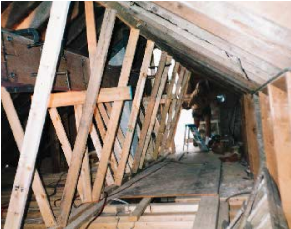
Before cutting away the peak of the existing roof, the authors built angled kneewalls on each side of the ridge. With horizontal 2x4s nailed across them, the kneewalls also served to support the built-up LVL beam while it was bolted together and lifted.
