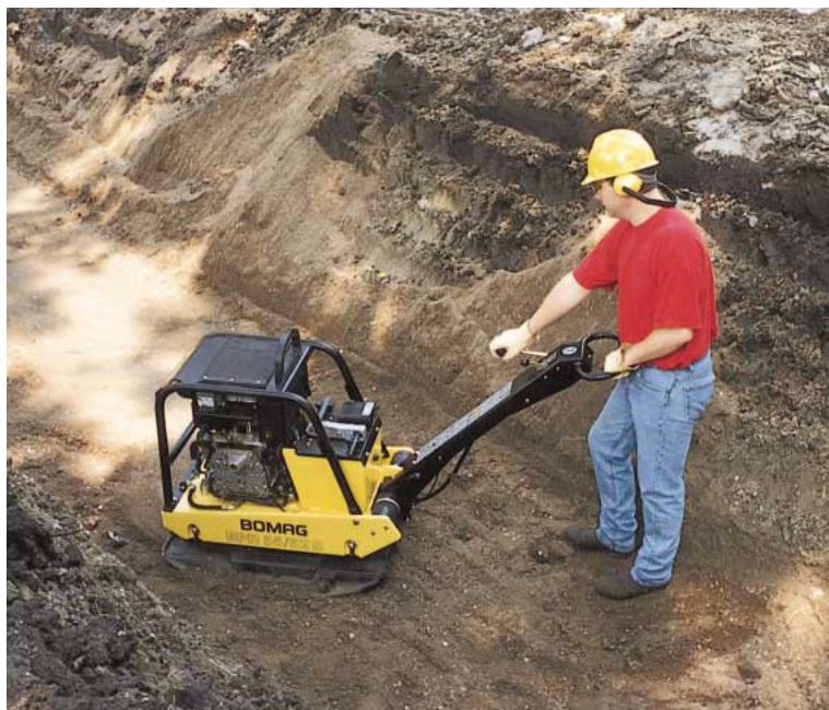
Figure 3. Lightweight, high-frequency vibrating plate compactors work best for fine to medium sands. Plate compactors are useful for trenches and other hard-to-reach areas.
