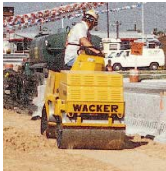
Figure 2. Smooth-drum vibratory rollers work best for compacting large areas of granular materials such as sands.
