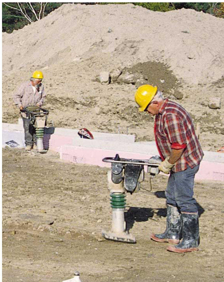
Figure 4. The kneading action of hand-held rammers compacts cohesive soils, and also works well on confined granular materials.
