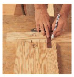
Use an adjustable square to tick off dowel locations on stiles and rails. Number or letter corresponding door parts.
