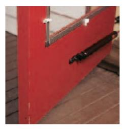
Readily available plastic or aluminum clips do a good job of holding the storm or screen panels in place.
