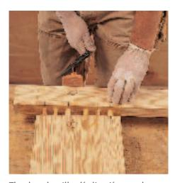
The dowels will self-align if properly centered and drilled. Use a pair of pipe clamps on a flat surface to glue up the door.
