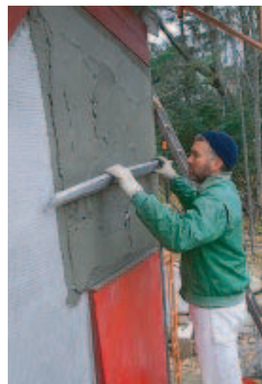
Figure 1. The brown coat is smoothed with a straightedge in preparation for the finish coat.
