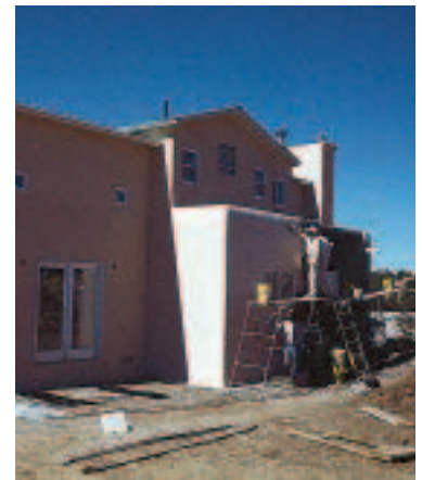
Figure 6. Working in the shadows is a good way to prevent rapid drying on a hot day.
