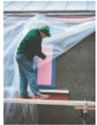
Figure 5. Covering stucco in cold or inclement weather extends the curing period and protects against a washout in case of rain.
