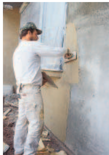
Figure 2. The \frac{1}{8} -inch-thick finish coat is applied with a trowel.
