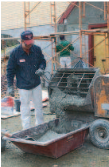
Figure 3. Close attention must be paid to mixing stucco to ensure a uniform and durable coating.
