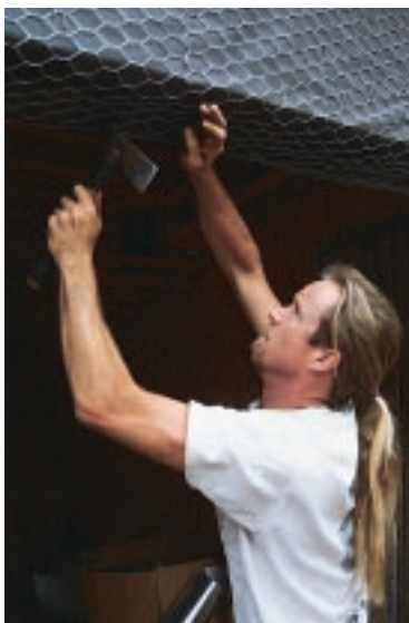
Figure 4. Careful lath and flashing installation sets the tone for a high-quality job.
