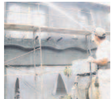
Figure 7. Spraying stucco in hot, dry, or windy weather prevents excessive evaporation.
