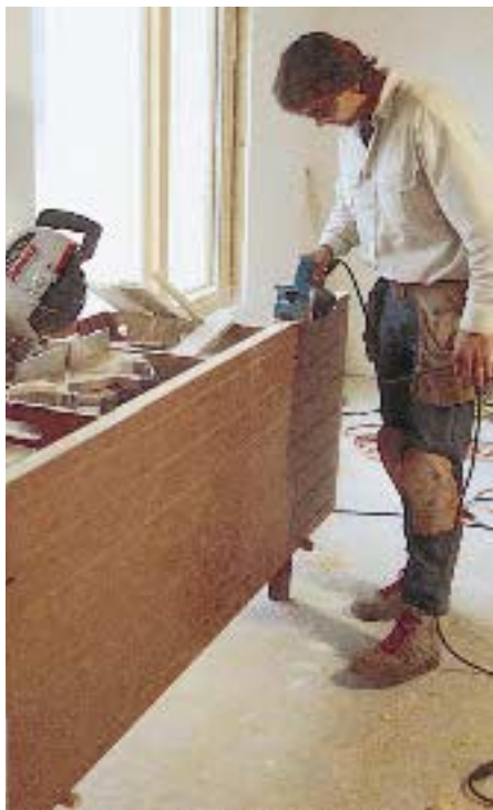
Figure 1. The author's crew use special workbenches to assemble jambs and hang doors on site. The benches hold door panels on edge at a convenient working height, and are equipped with all the tools and jigs needed to hang doors and install hardware.
