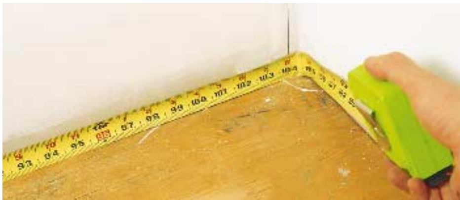
Figure 5. Precutting all baseboard speeds installation. To get accurate dimensions, trace the outline of the base molding on the wall (top) and measure to your mark (above). This is the short-point of the miter that will guide the coped corner cut.
