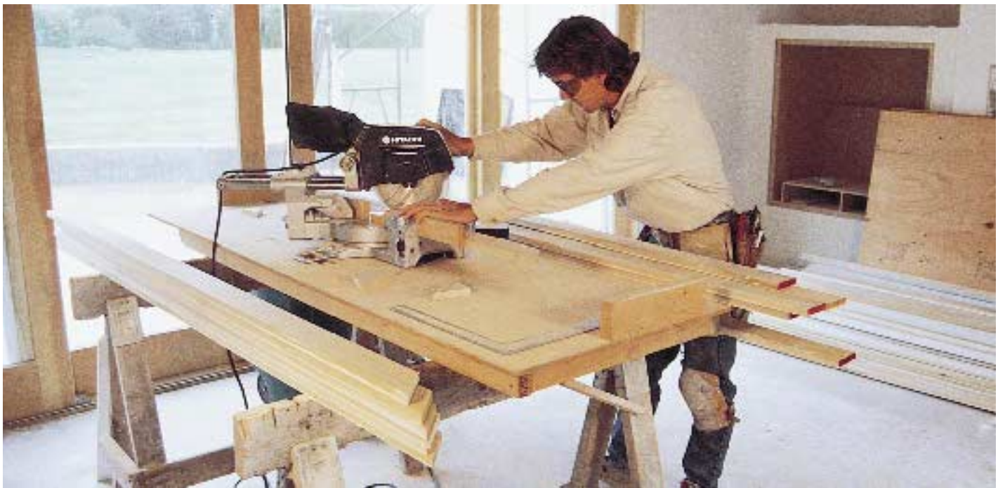
Cutting casings for ten doors at a time greatly speeds production.
