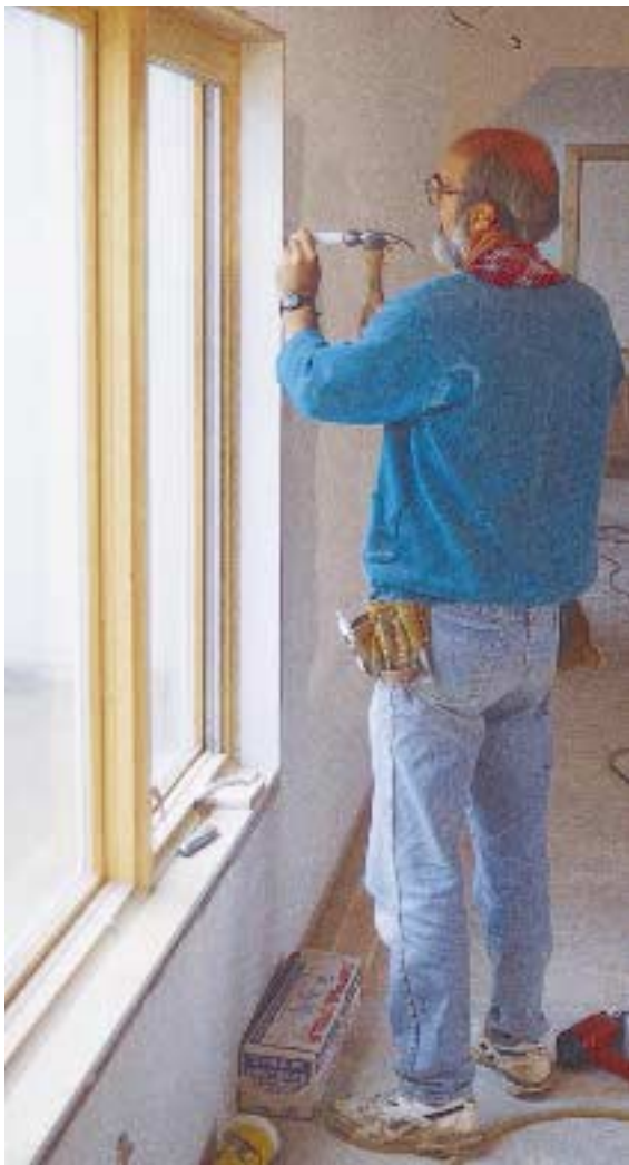
Figure 4. To speed installation of extension jambs, pre-assemble them on a workbench, then shim and nail to the jack studs just like a door jamb.
