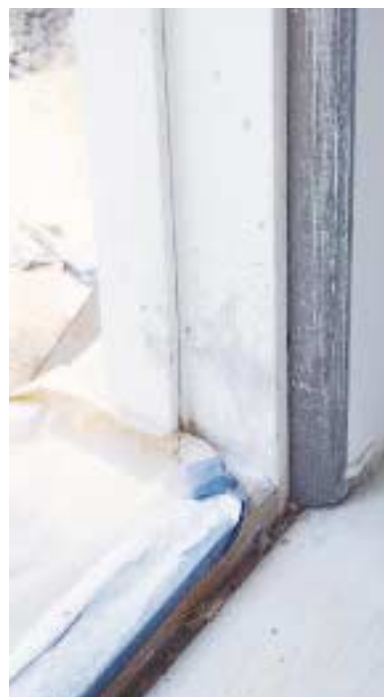
Figure 2. The author uses either L-bead or bullnose corner bead (photo) for a trimless, Mediterranean look. To ensure a clean reveal, he cuts a shallow kerf in the edges of the jambs, into which one leg of the bead is inserted (illustration).
