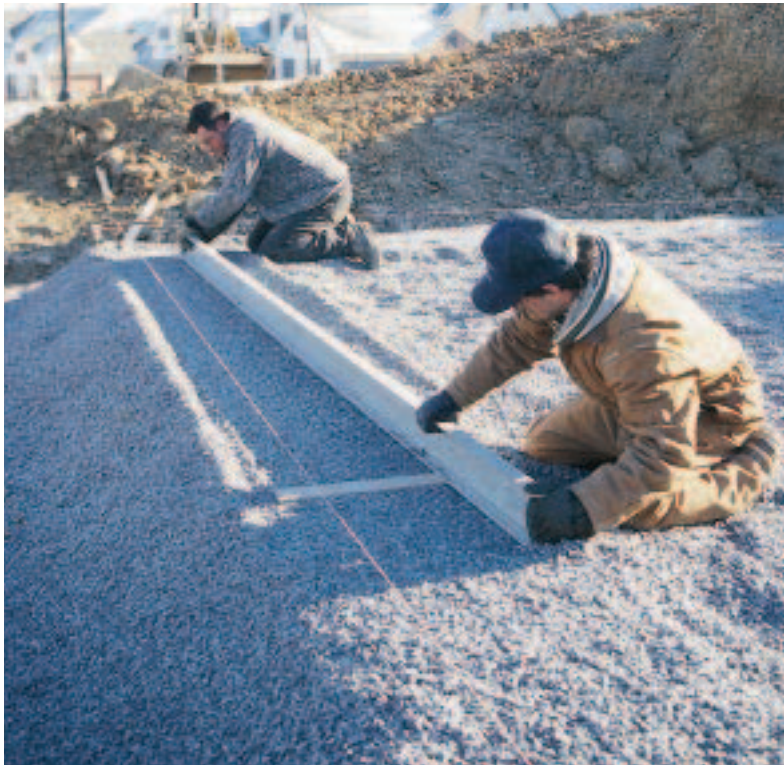
Figure 1. In areas where the panels will sit, the gravel is compacted with a vibratory plate compactor, then accurately leveled using a magnesium straightedge.
