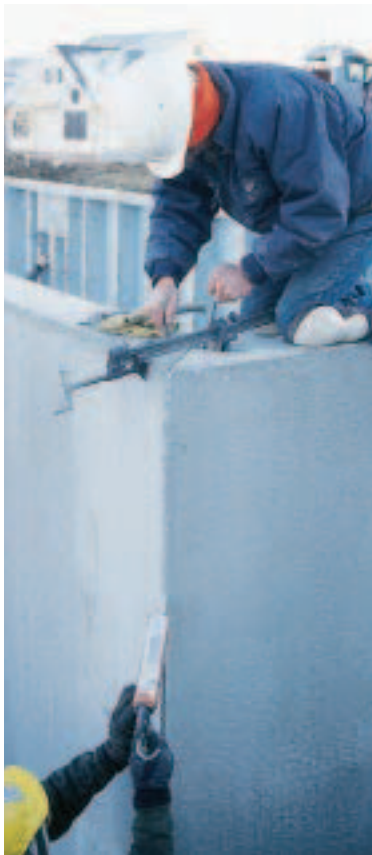
Figure 2. Half-inch bolts, inserted through cast recesses, fasten the panels together at the top and bottom plates (left). A bead of urethane sealant is applied to the butt joints, and after the panels are drawn up tight, the joint is caulked again on the interior and exterior (above).
