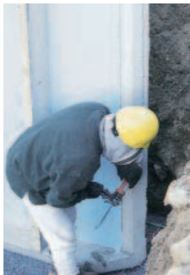
Figure 2. Half-inch bolts, inserted through cast recesses, fasten the panels together at the top and bottom plates (left). A bead of urethane sealant is applied to the butt joints, and after the panels are drawn up tight, the joint is caulked again on the interior and exterior (above).
