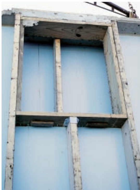
Figure 3. Window openings are framed with treated 2x8s. Sizes and location must be specified when the panels are ordered.
