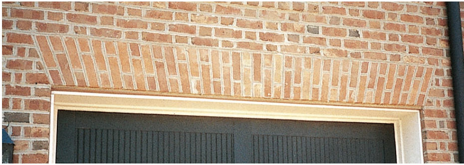
Figure 3. With a correctly installed factory-made jack arch (photo, above), the center brick is perfectly vertical, while the bricks to the left and right are tapered and skewed symmetrically at an ever-increasing angle. Note that the top and bottom of the arch are perfectly parallel and that the height of the arch matches the brick coursing. “New concept” arches (drawing, at left) use a keystone and a series of bricks all cut with exactly the same shape. They lack the authenticity of a true arch kit, but are less expensive.
