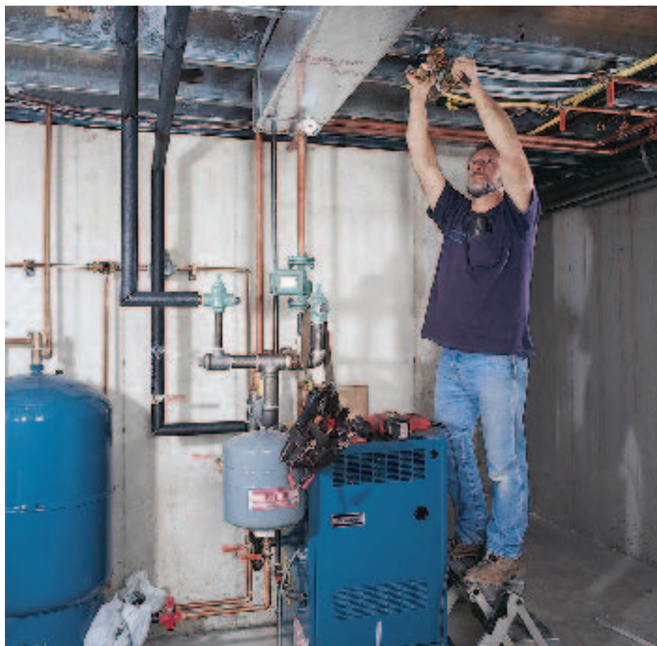
A mechanic connects floor manifolds to the PEX tubing that supplies heat to the slab on the first floor.
