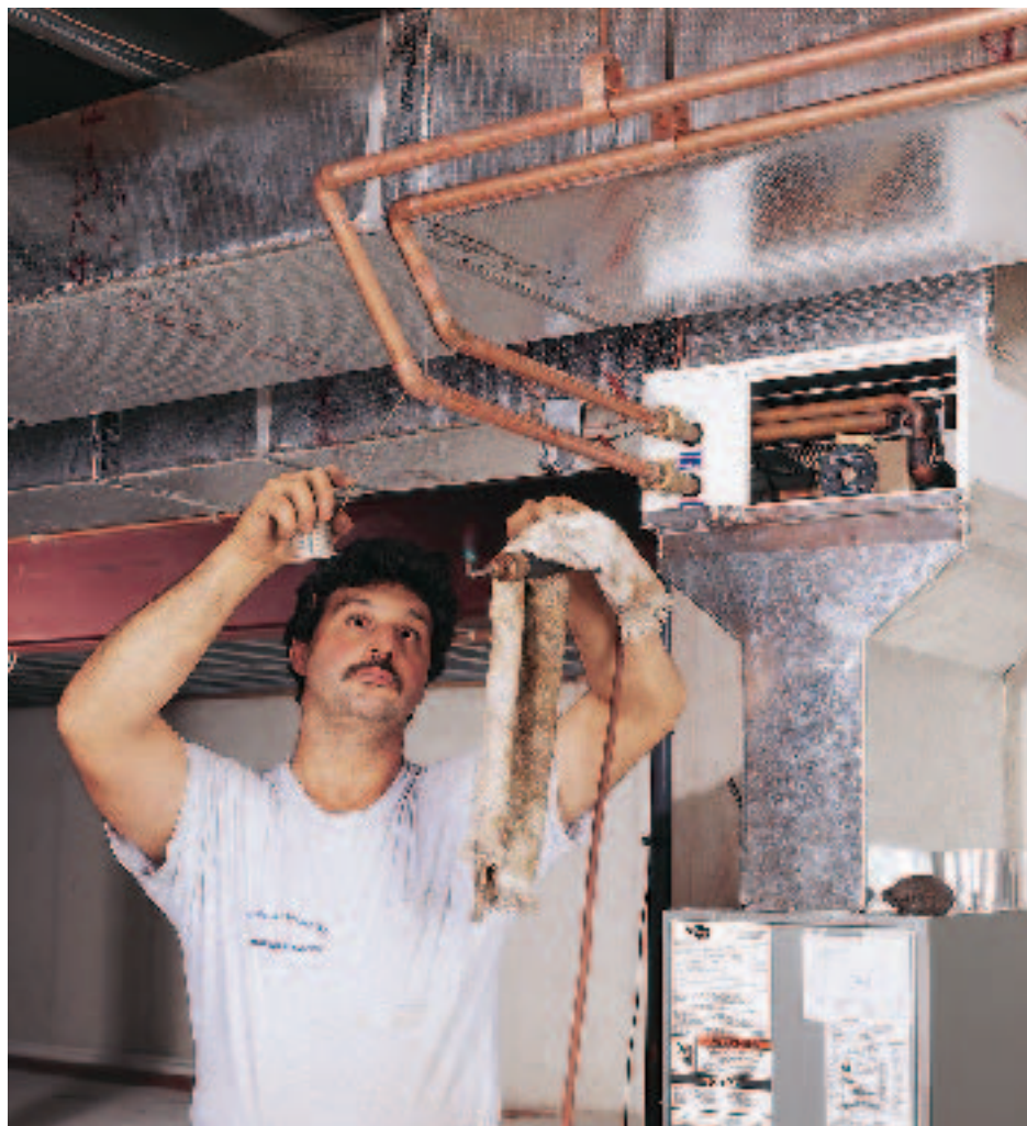
An hvac mechanic solders the hot water supply and return lines at the heating coil. The author prefers separate heating coils to built-in units because they allow for more accurate sizing.
