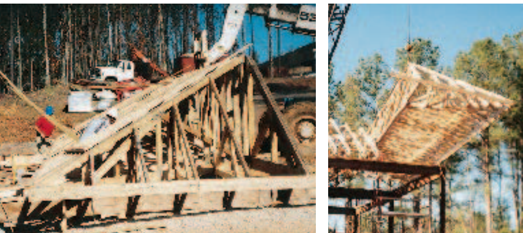
Figure 2. Framing truss roofs on the ground reduces dangerous work on the roof. The hip end shown here, part of a large commercial job, was completely framed on the ground (left), then craned into place (right). On residential work, the author usually installs the king hip girder and hip jacks on the roof.
