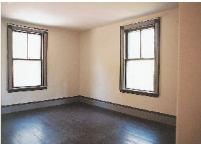
Figure 1. While the room was large enough for a bath (left), the existing window placement and direction of floor joists somewhat limited the choice and placement of the fixtures. Putting the tub in one corner (right) and the toilet on the wall opposite allowed the drain lines to share the same joist bay, limiting demo work and plumbing costs.
