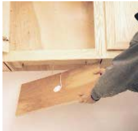
Figure 2. The pucks mount neatly in holes in a false bottom panel, which is attached to cleats in the cabinet's bottom recess. The panel removes easily for maintenance.
