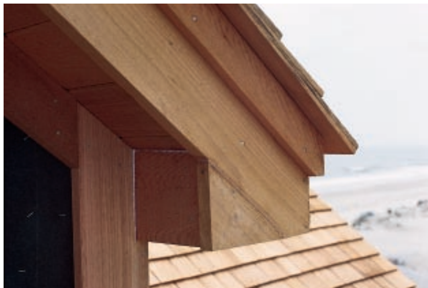
Figure 3. A 1x2 trim board held ¾ inch higher than the roof sheathing hides the edge of the Cedar Breather.
