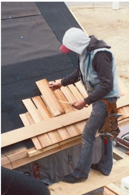
Figure 2. Tacking a 1x6 “exposure guide” flush with the bottom of every shingle course makes it easy to position and fasten the next course.
