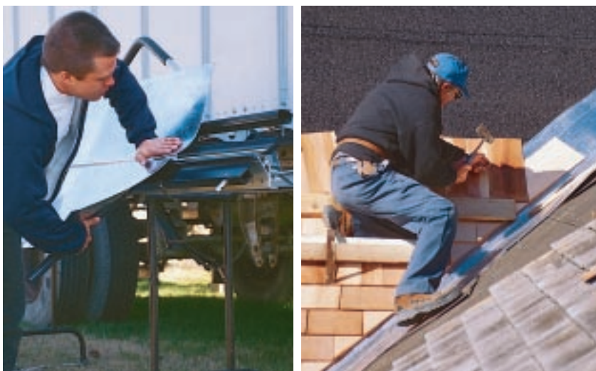
Figure 4. The author's crew forms the lead-coated-copper valley flashing with a 10-foot brake (left). The inverted V in the center of the flashing directs runoff down the valley. When attaching valley shingles, nails are held at least 12 inches from the center of the valley (right).
