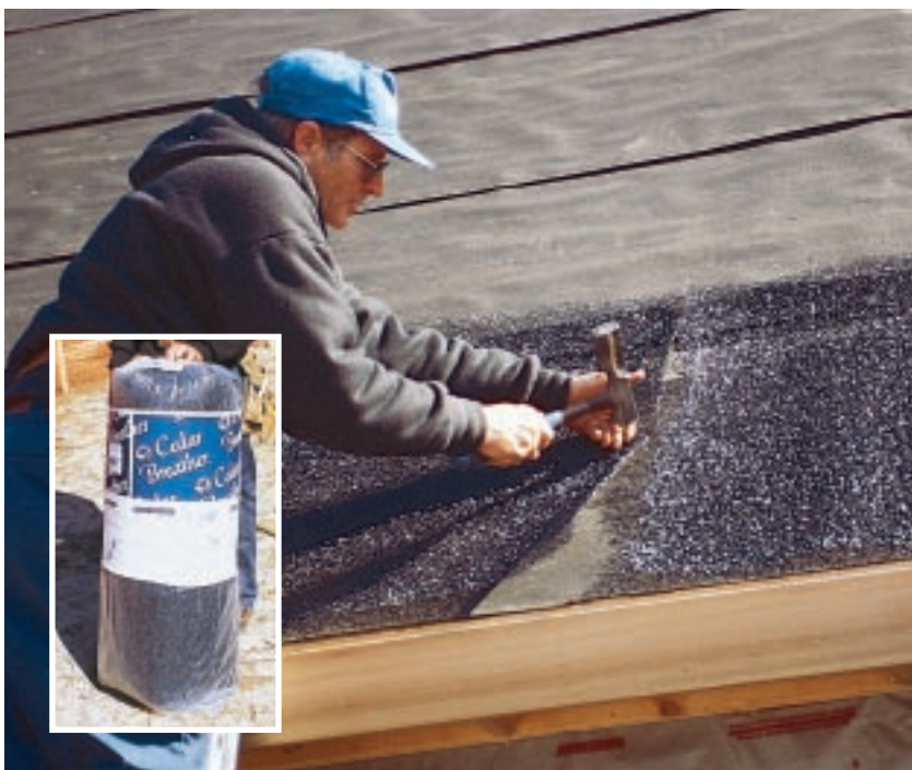
Figure 1. A 3/8-inch-thick layer of Cedar Breather (inset) laid over solid sheathing and felt paper allows the wood shingles to dry from underneath.
