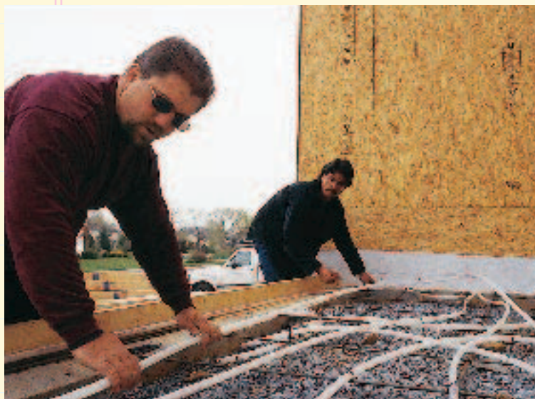
Hvac contractor Joe Giandalia (right) and a helper install radiant tubing for a snowmelt system in Lancaster, Pa. New materials have brought the systems to the $2.50- to $3-per-square-foot range.
