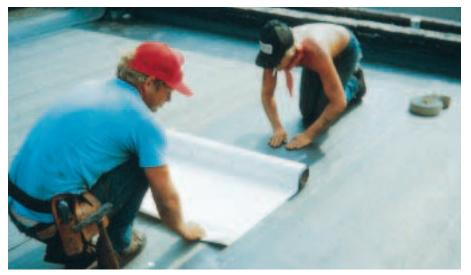
the roof. A 3x34-foot roll of Kwik Ply weighs about 40 pounds and can be handled and installed by one person. The material comes with a limited 10-year warranty and costs around \$3 per square foot.
