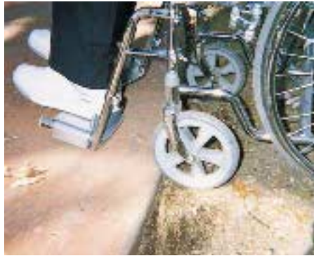
A wheelchair operator can be catapulted from his seat when the chair's front wheels strike this small lip.
