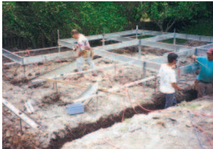
Inventor Michael Butler and his crew assemble a floor frame from lightweight steel C-channel (left). Perimeter forms are hung from the suspended frame (below).
