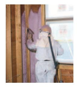
Corbond's trademarked lavender color allows applicators to monitor product consistency by eye. The medium-density foam has an insulation value between R-6 and R-7 per inch, and good air-sealing properties.
